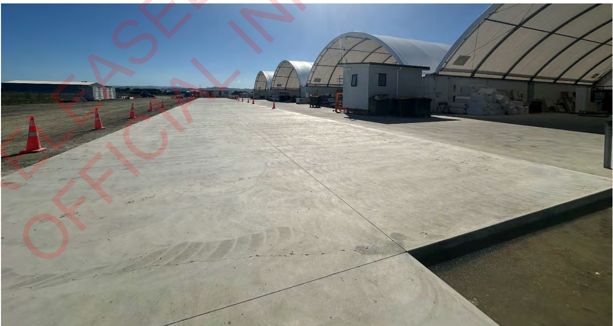
Below image: Concrete completion as at 26 January 2024
