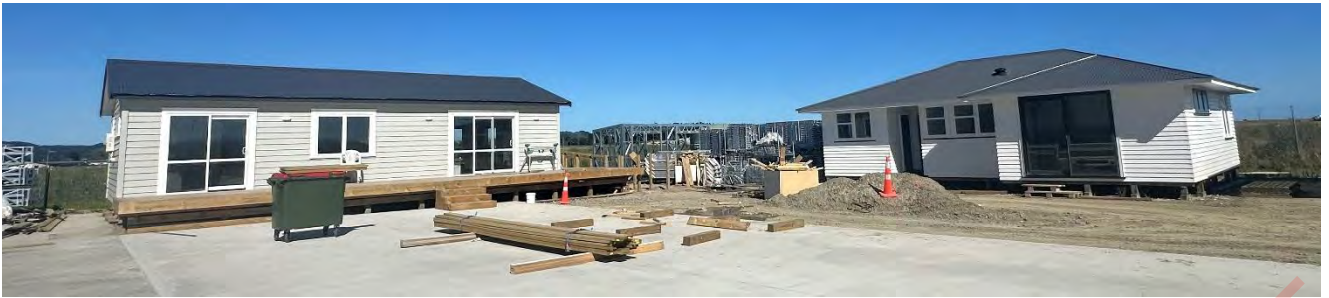
Above image, new office and pre-loved home. Pre-loved remedials are progressing well, as per above image.
