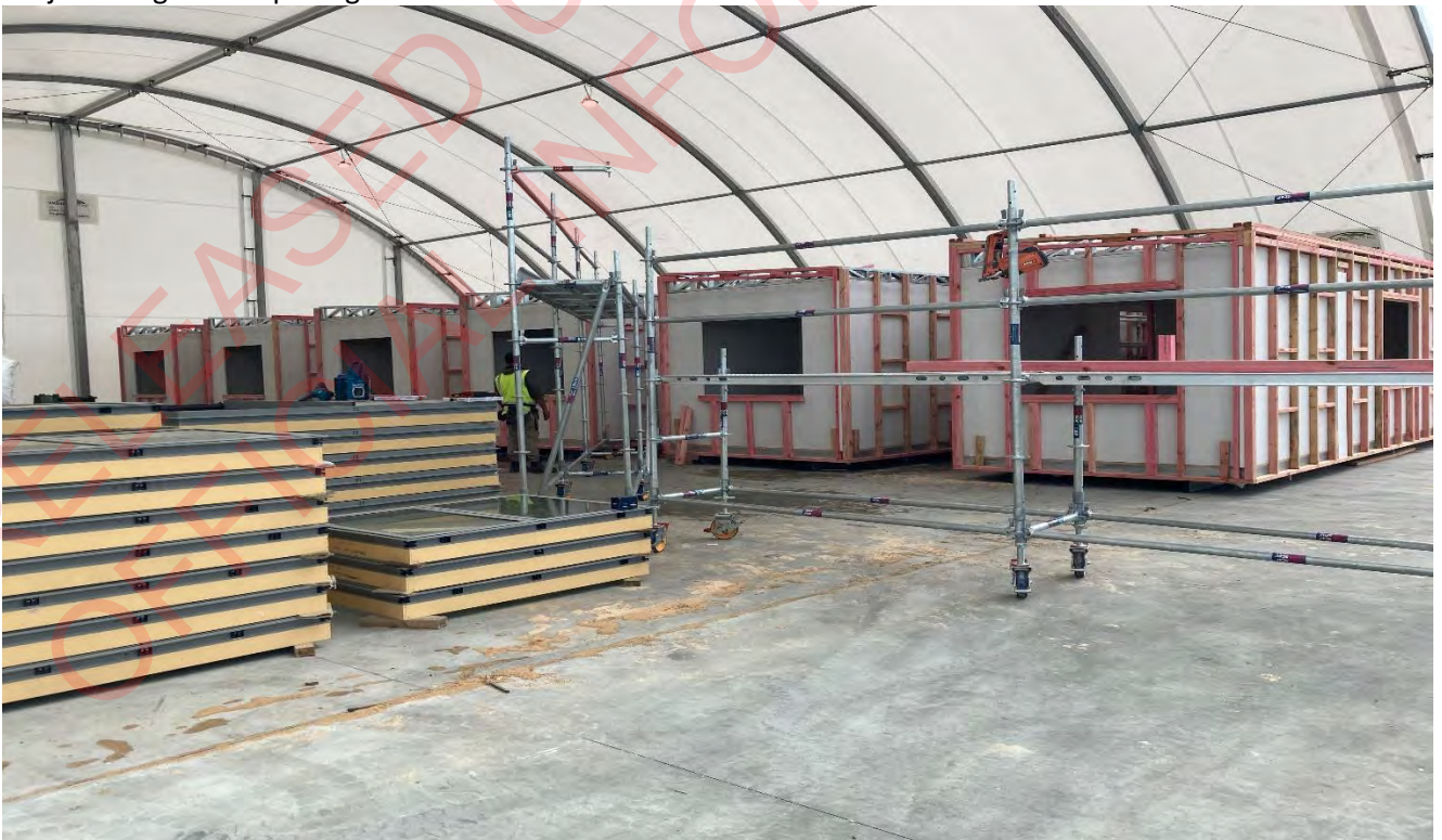
Image above: Te Wharau o Hineakua, Toitū Tairāwhiti Builtsmart – 6 Whare Āwhina in build progress.
