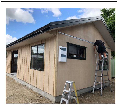
New social housing flats for Huia Street being built off-site
