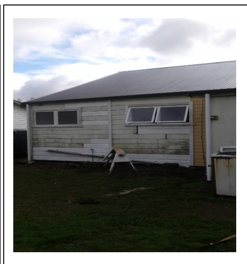
Old roof compared to new roof
