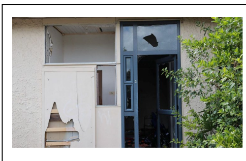
Old Huia Street flats now demolished
