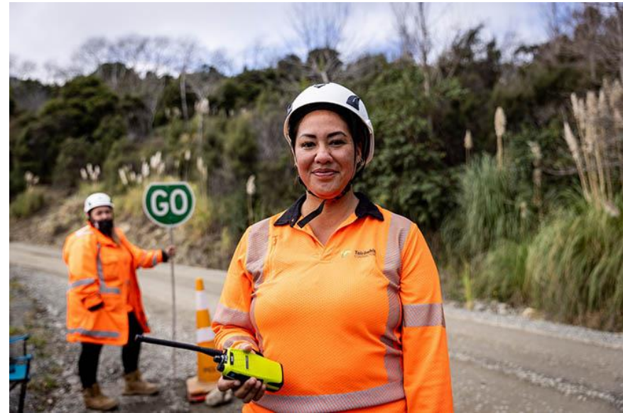
This is Kat from (Ruatōria based) Tairāwhiti Contracting who successfully secured a government procurement contract to repair the cyclone-ravaged East Coast State Highway 35 with another contractor.
