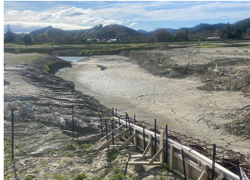
Wi Pere Finishing Farm, adjacent to the Waipaoa awa about 20 kilometres north of Gisborne, had over half of its 870 hectares inundated with sediment and debris when the Waipaoa stop bank broke in the wake of Cyclone Gabrielle in February 2023.
